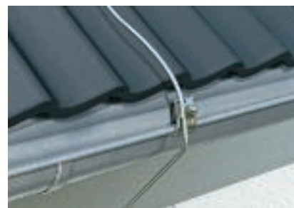
Conductor, connected with gutter clamp
